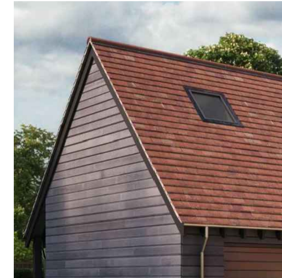
timber cladding with tiled roof
