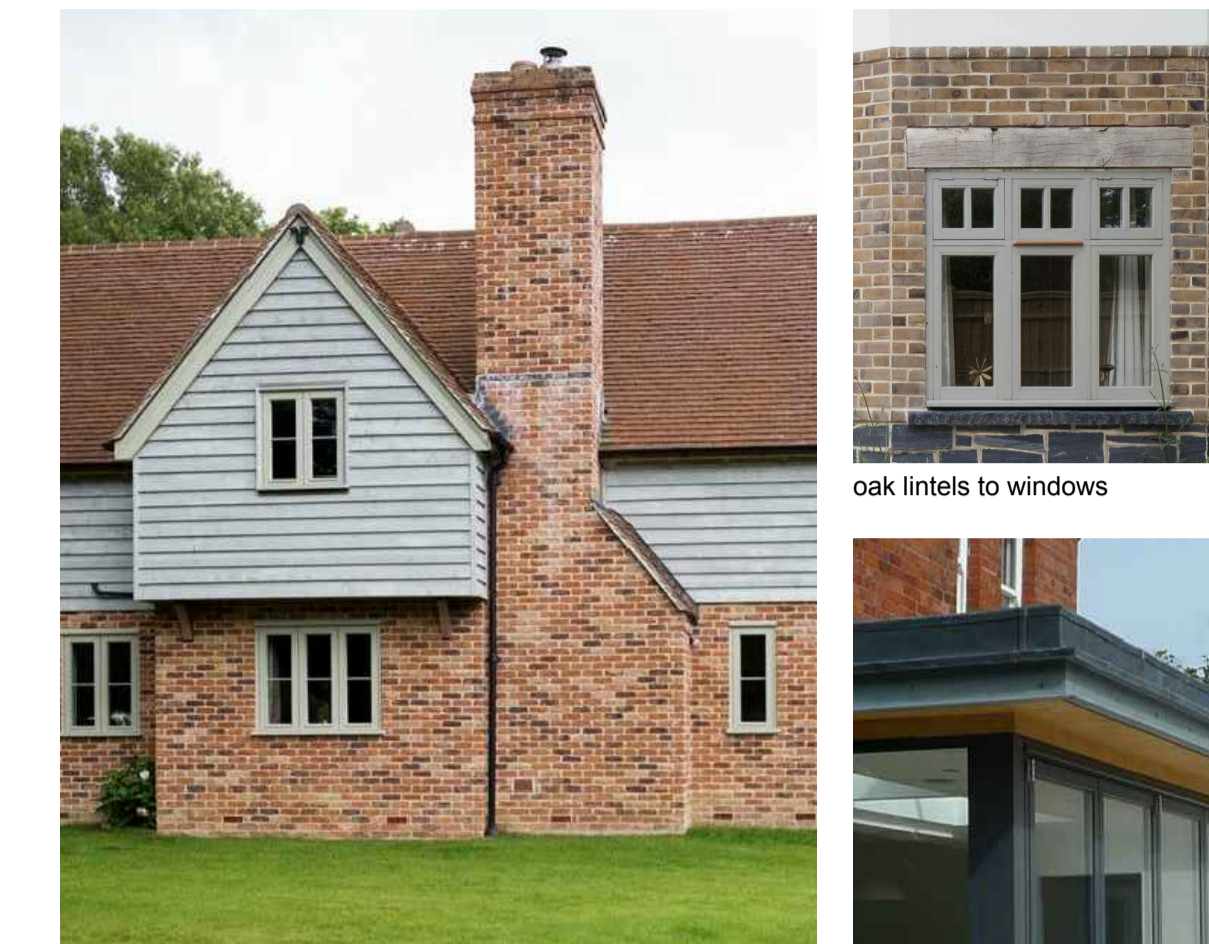
juxtaposition of timber cladding, brickwork and clay tile roof
